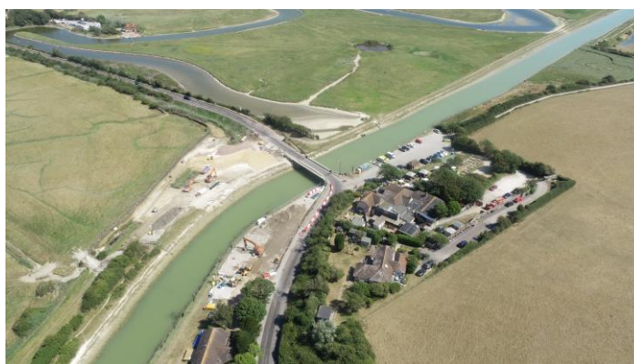
Site preparing for piling works at Exceat Bridge
