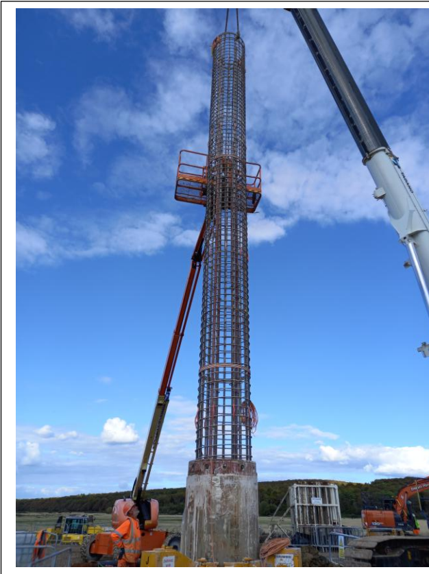
Bored piling progressing on the west side
